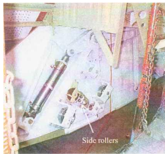
Figure 13. Inboard Flap rollers (flap removed)
